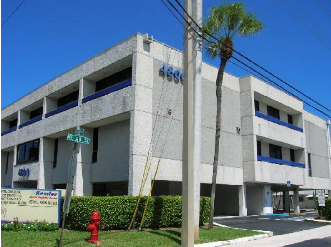
Front & Garage View
